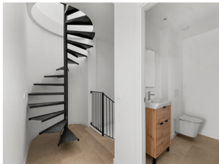
Access to the roof terrace
