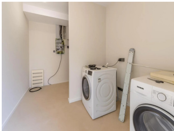
Separate utility and laundry room
