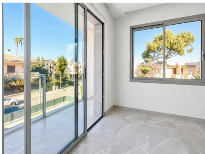
Third bedroom on the upper floor
