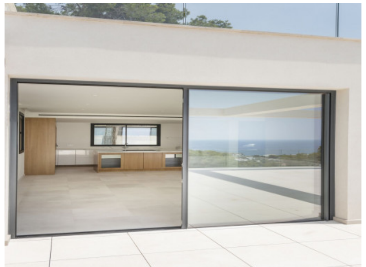
View from the outside
