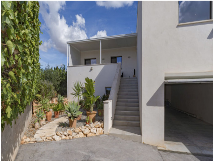
Entrance to House and Garage
