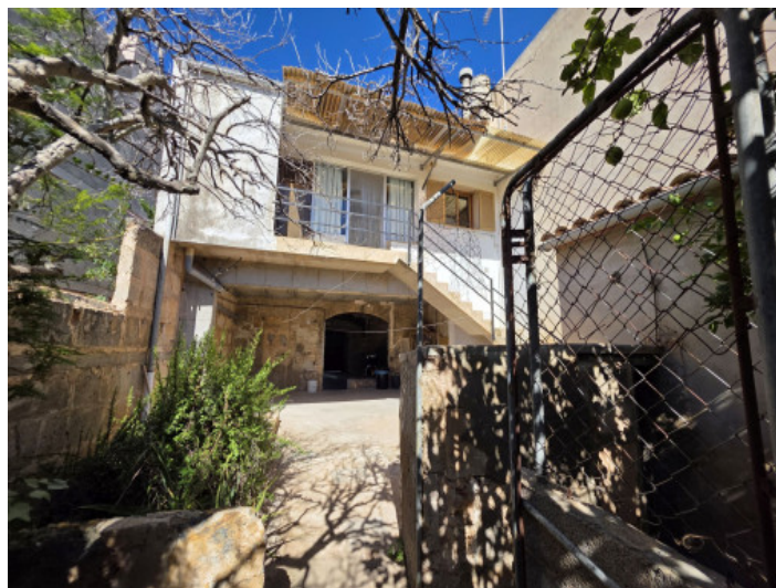
View of the house from the garden
