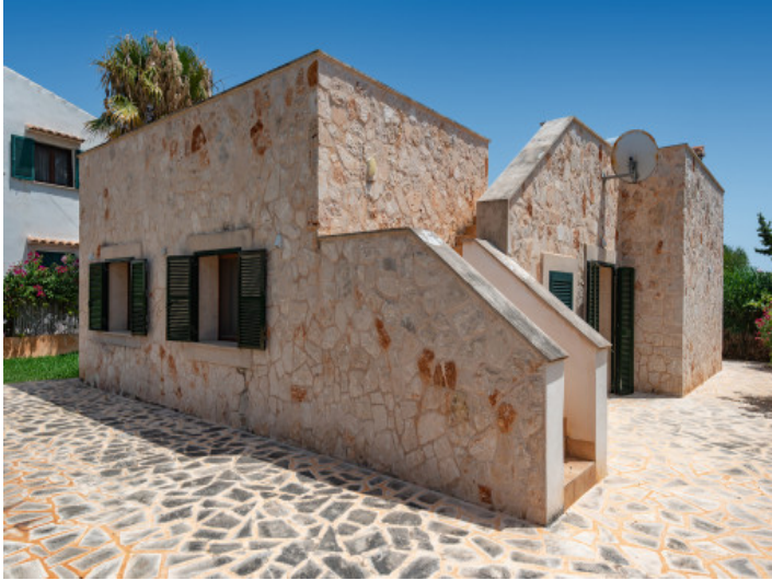
Stairway to the rooftop terrace
