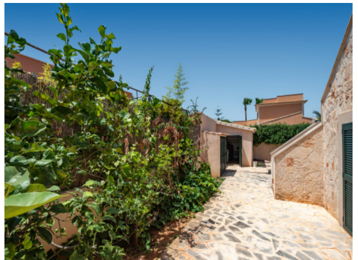
Garden surrounding the house, with the stairway to the rooftop terrace on the right
