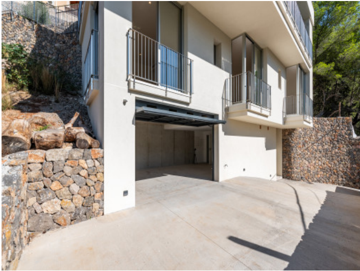
Access to the garage
