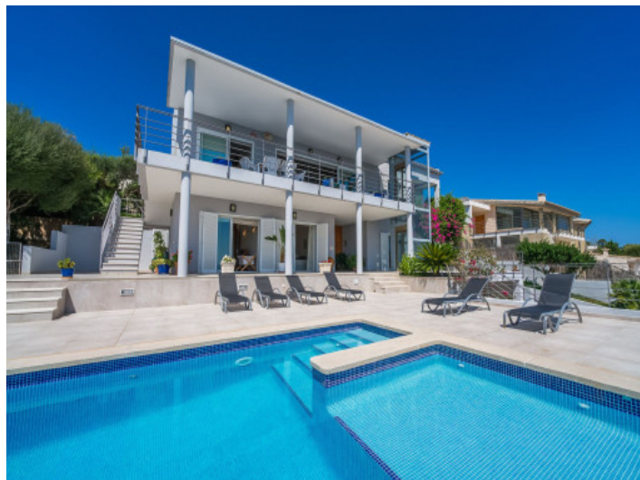
Exterior view and pool area
