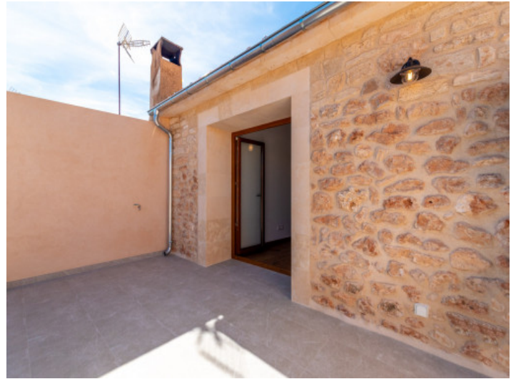
View of the balcony
