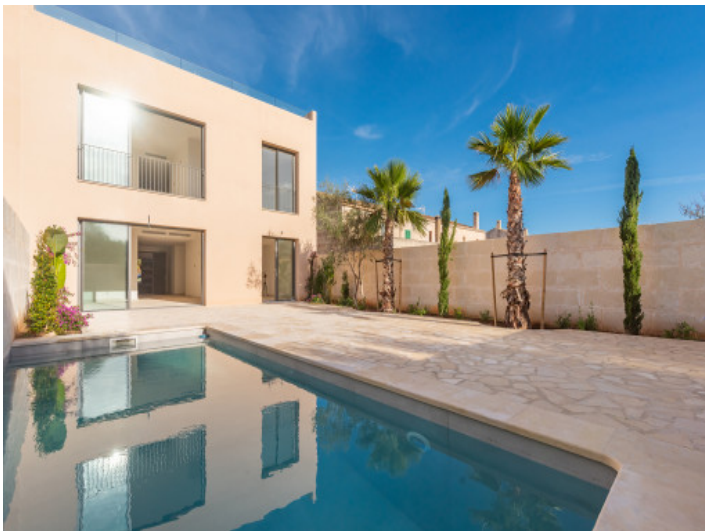
Modern town house with pool in Ses Salines
