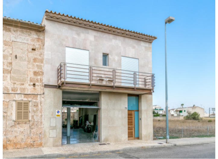
Exterior view of the town house
