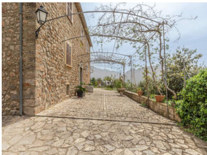
Terrace and exterior view
