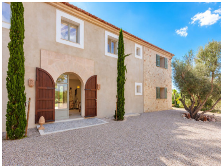
Frontside with driveway
