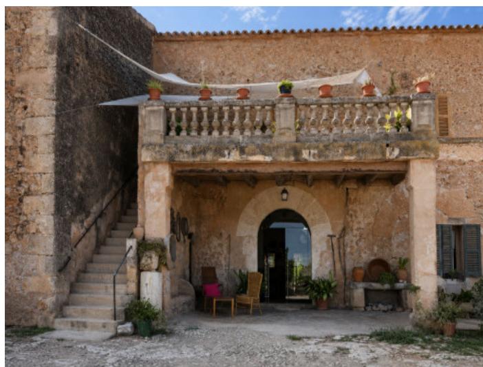
Main Façade with Terrace
