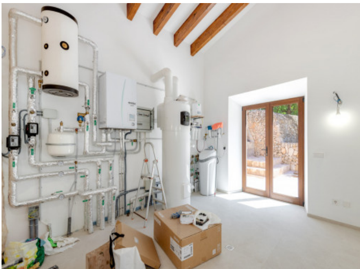
Storage and utility room
