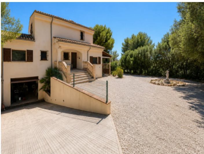
Driveway with direct access to the garage
