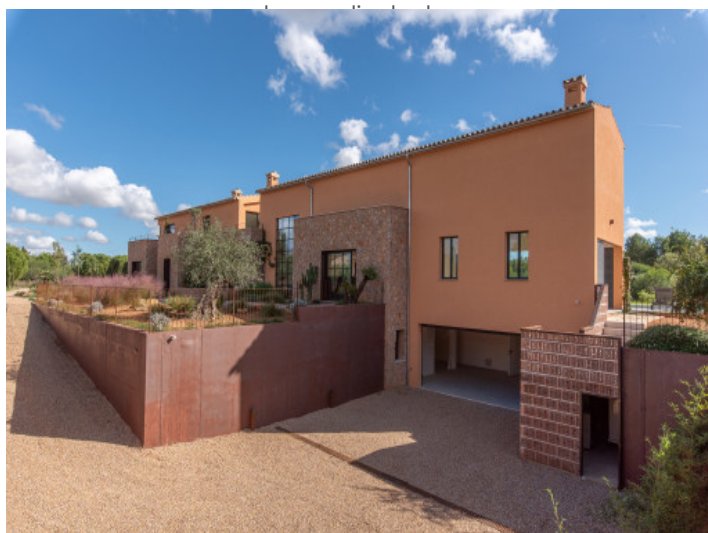
Access to the garage
