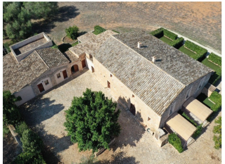
Main House with 10 Suites
