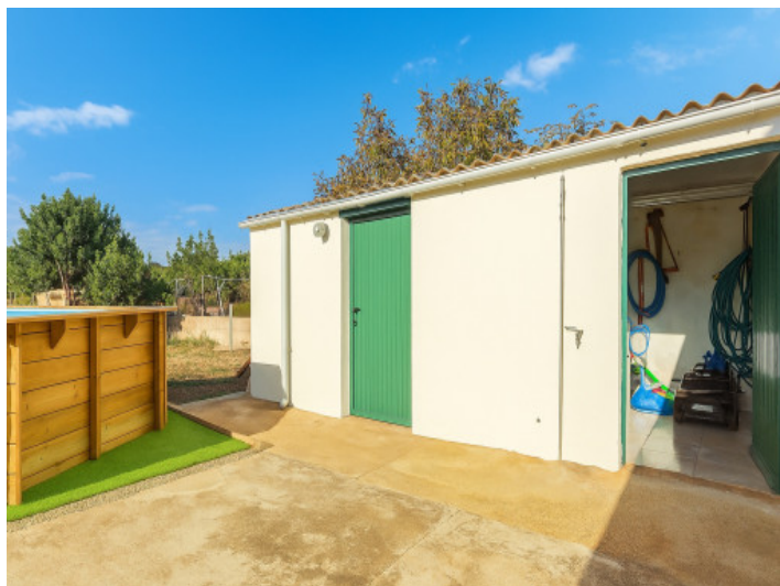
The swimming pool and the annex building
