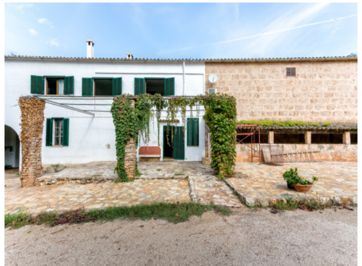
Front view of the rustic finca
