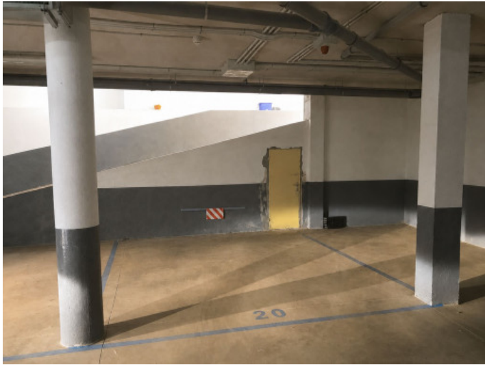
Large underground parking space with adjacent storage room
