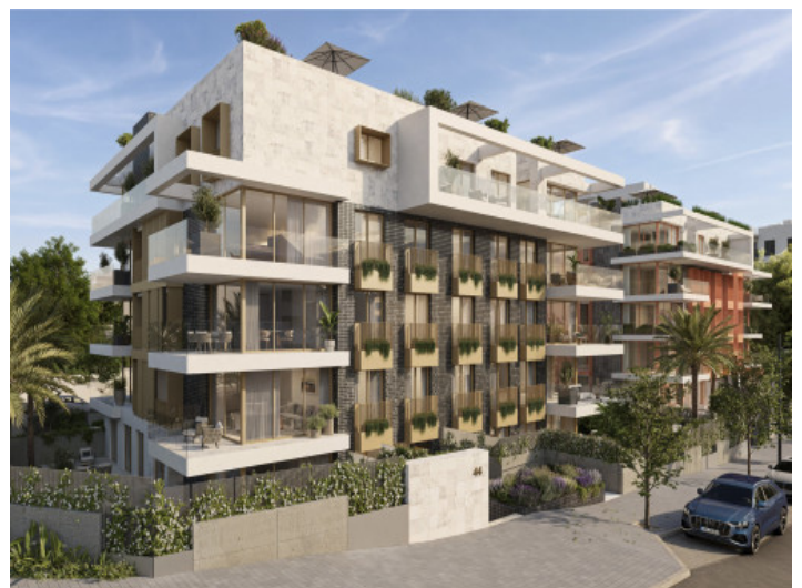
Facade and entrance
