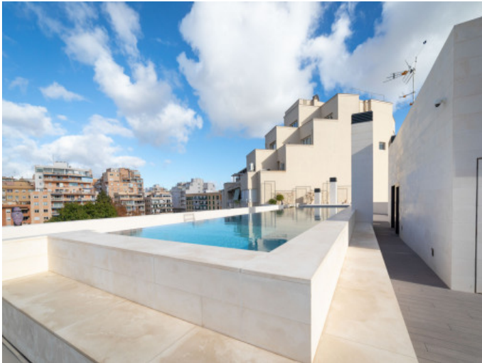
Pool is surrounded by a terrace
