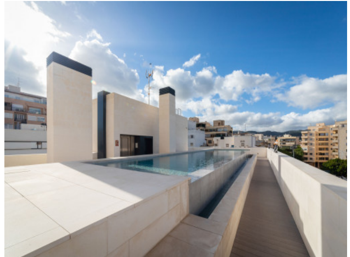
Roof terrace with pool
