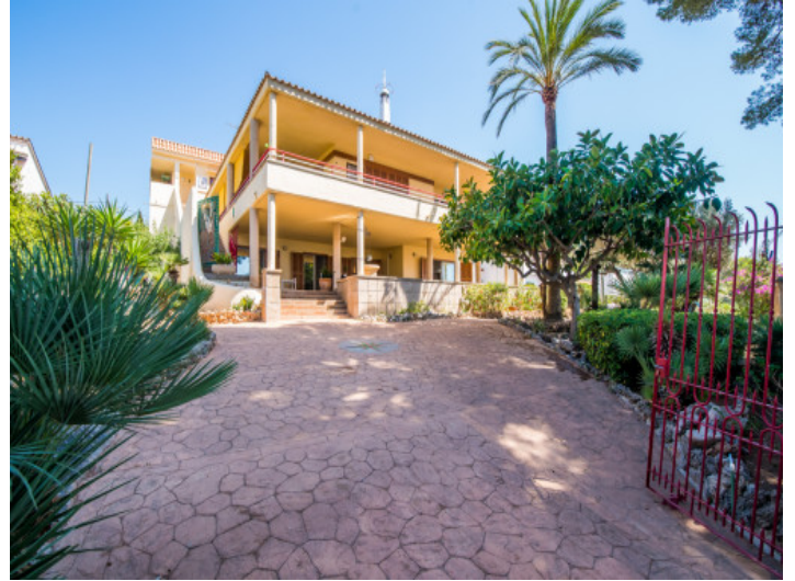
Access to the house
