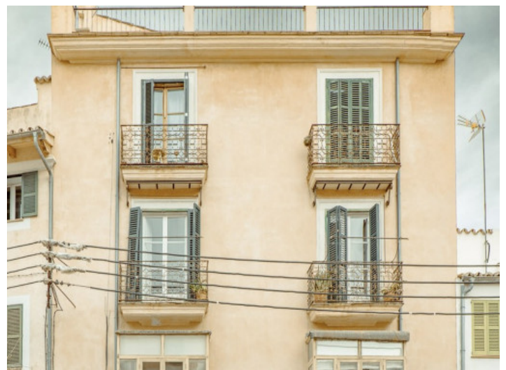
View to the building
