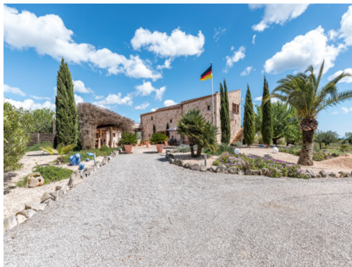
Access to the property
