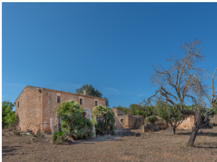
Historic finca-property requiring renovation in Sant Llorenç des Cardassar
