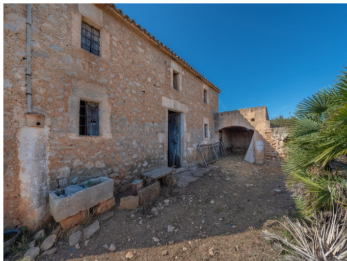
Facade and access
