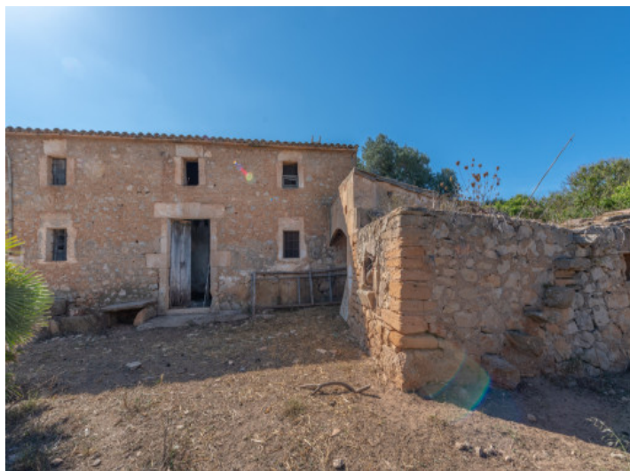
Facade and access
