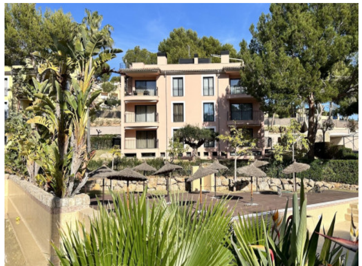
Facade and garden area
